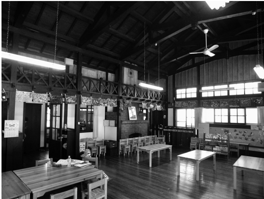
Figure 4. The spacious classroom in the kindergarten section Note: The Western-style roof truss and observation gallery can be seen.
